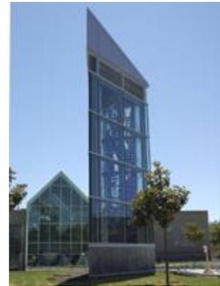
*(Above and below) The new underground library at Regent College is heated and cooled by a radiant system. Air is exhausted from the 30,000-square-foot library through a 40-foot-high wind tower on the roof, requiring only infrequent use of electric fans. (KEN MCALLISTER/REGENT COLLEGE)*
